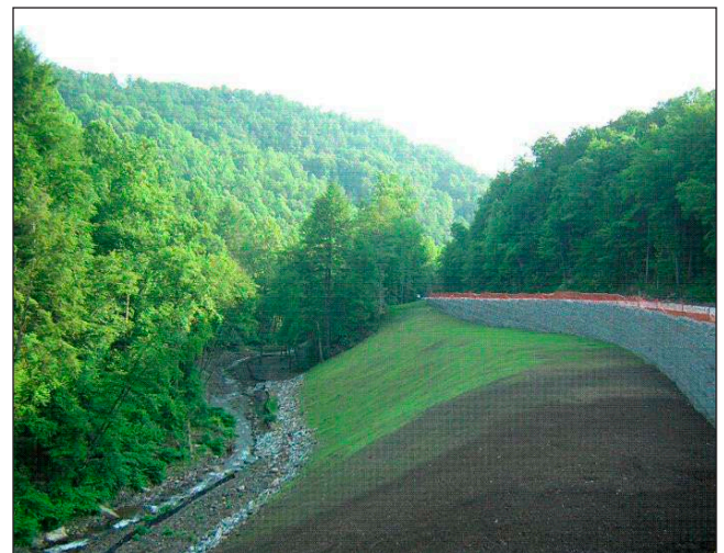
Figure 3 Establishing vegetation in a compost blanket
