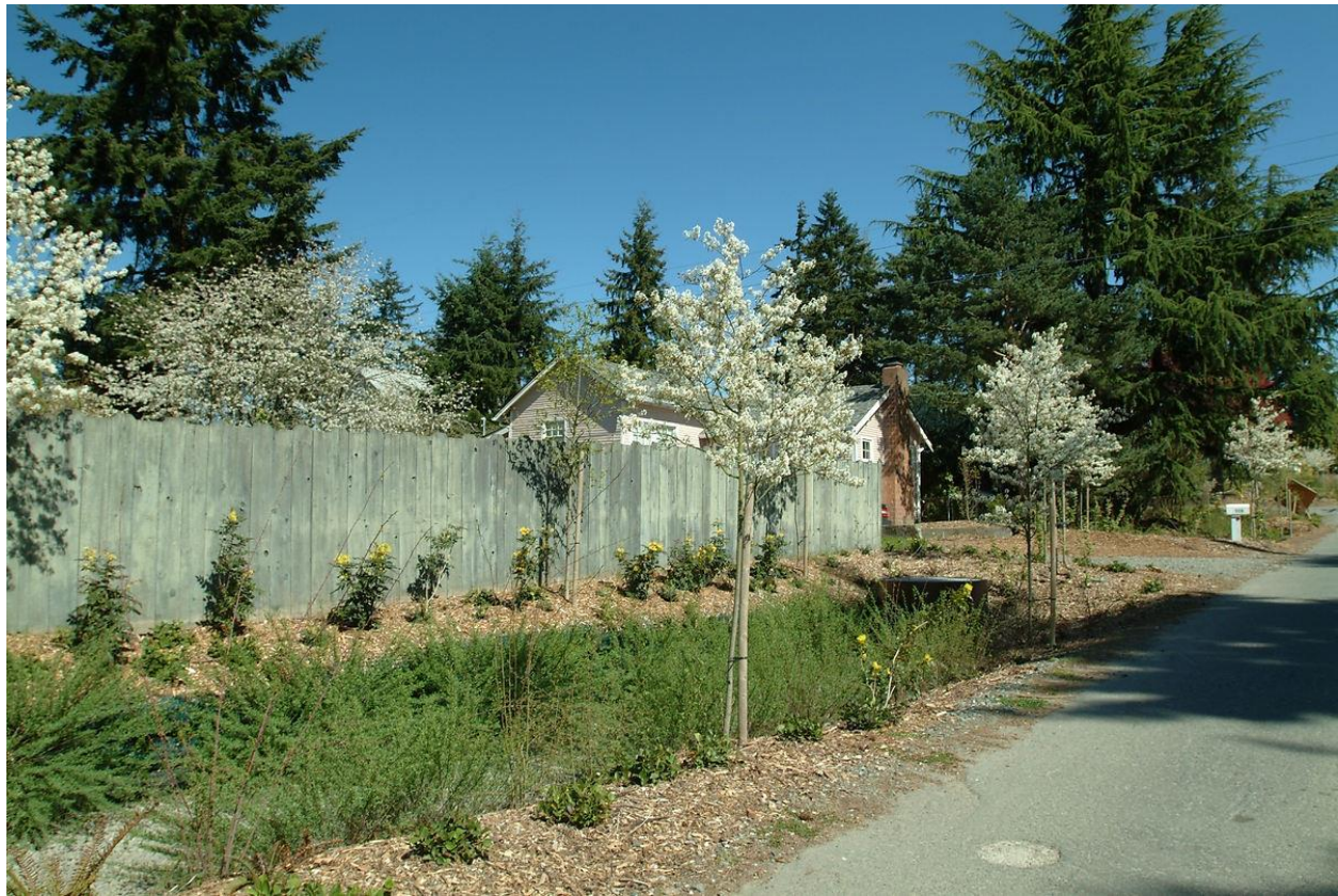
Figure 14. Compost-amended bioretention cascade along a residential street in Seattle, WA, with mulch, compost, plants and trees to support stormwater capture and filtration.
