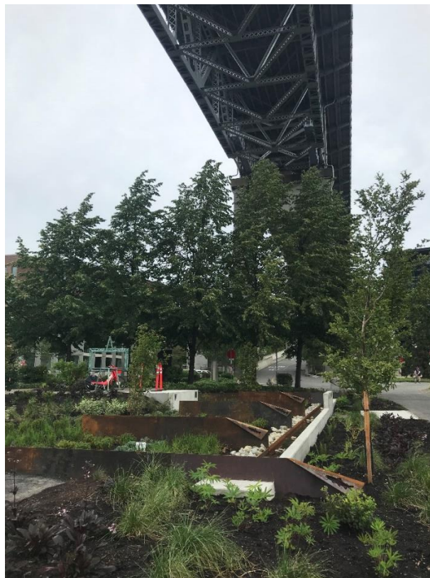
Figure 10. Green infrastructure for filtering stormwater coming off a bridge in Seattle, WA. Photo courtesy of Seattle Public Utilities.
