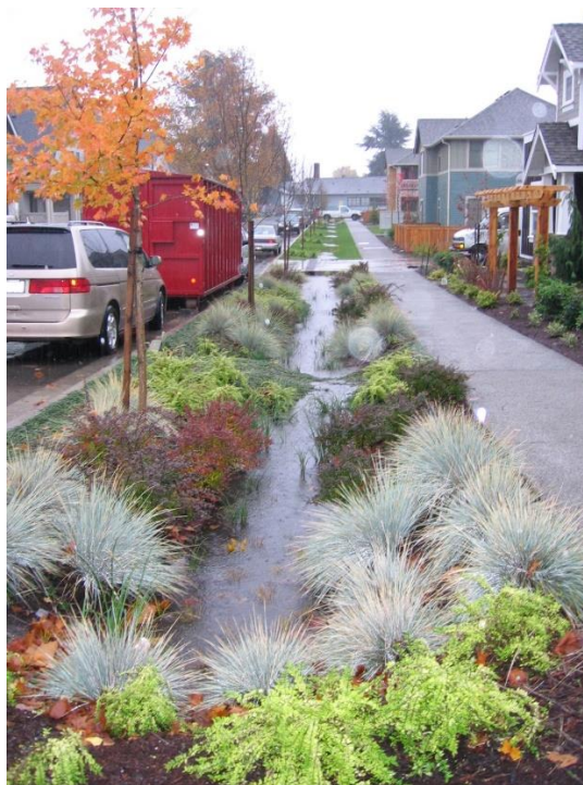
Figure 11. Street-side bioretention swales with compost-amended soils, across an area of 34 city blocks in Seattle, WA. Photo courtesy of Seattle Public Utilities.
